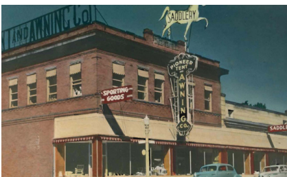
Integrated historic signage
