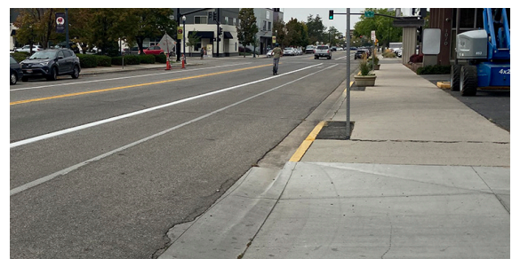
Needed curb and sidewalk repair
